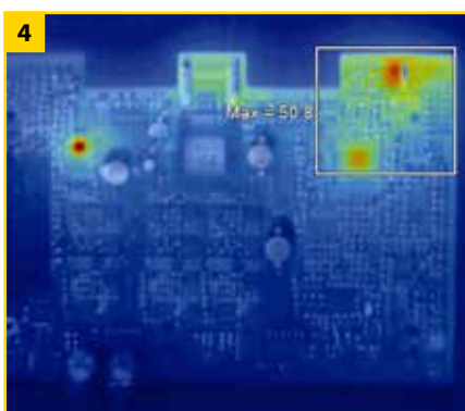
Badly soldered or faulty components on pcb's
