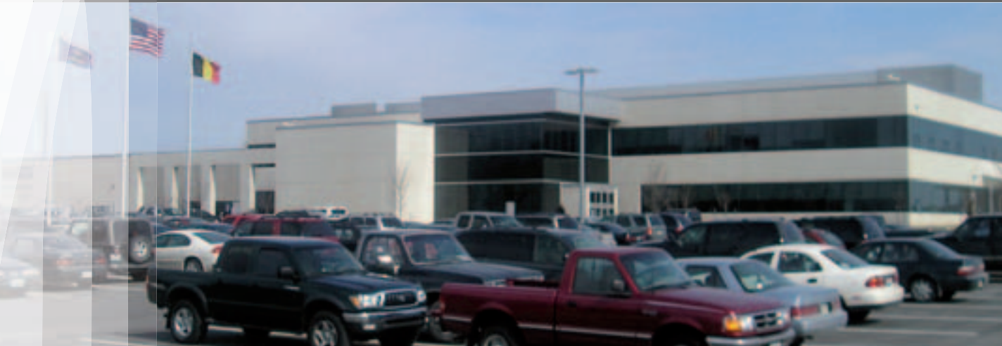
SMH Headquarters for the Americas, Olathe, Kansas (USA)
